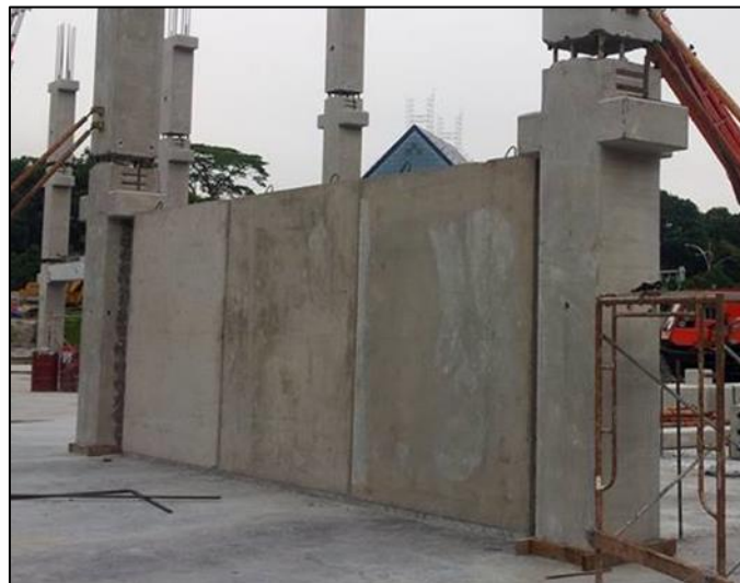
Figure 10. Precast non-load bearing wall
