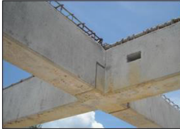
Figure 22. Beam to beam connection using the nib at the primary beam
