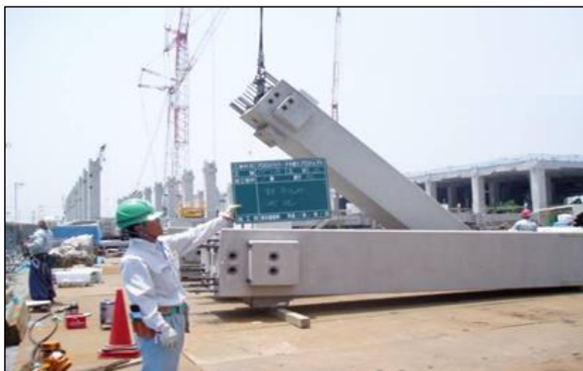
Figure 4. Lifting a precast concrete column component for erection and installation
