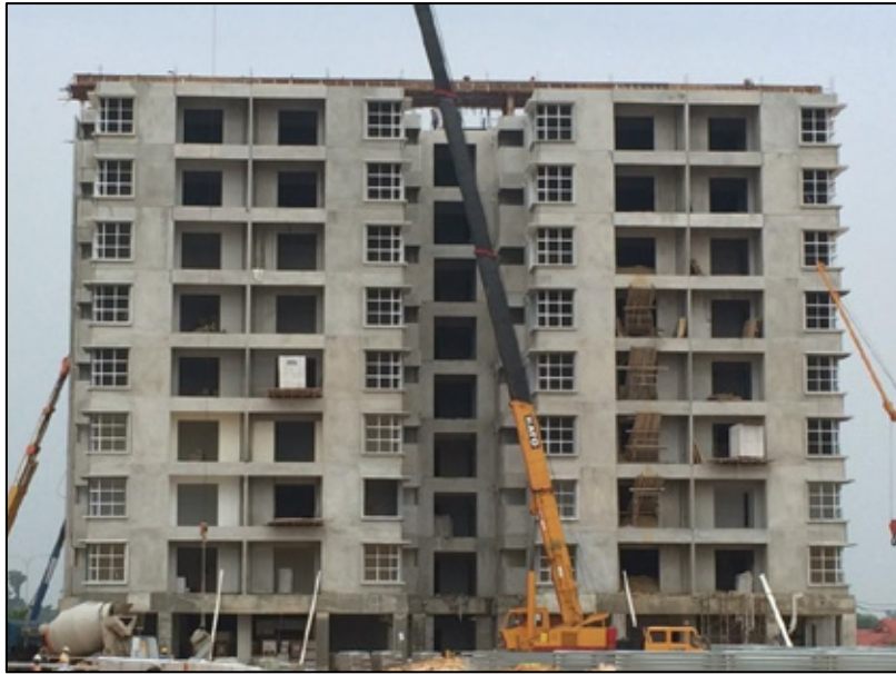
Figure 6. Quarters building using a load-bearing wall system
